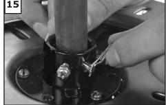
Insert downrod into yoke on top of the Fan Body. Align the hole in the Downrod with the hole in the Yoke. Insert the Pin through the Yoke and Downrod until the point appears on the other side. Install the Keeper Pin
